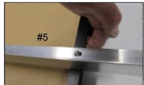
the bolts in the holes provided from underneath facing out (Photo #5) and tighten on the flange nut. It is important that the flange nut bears against the rail and not the panel frame, Photo #6.
